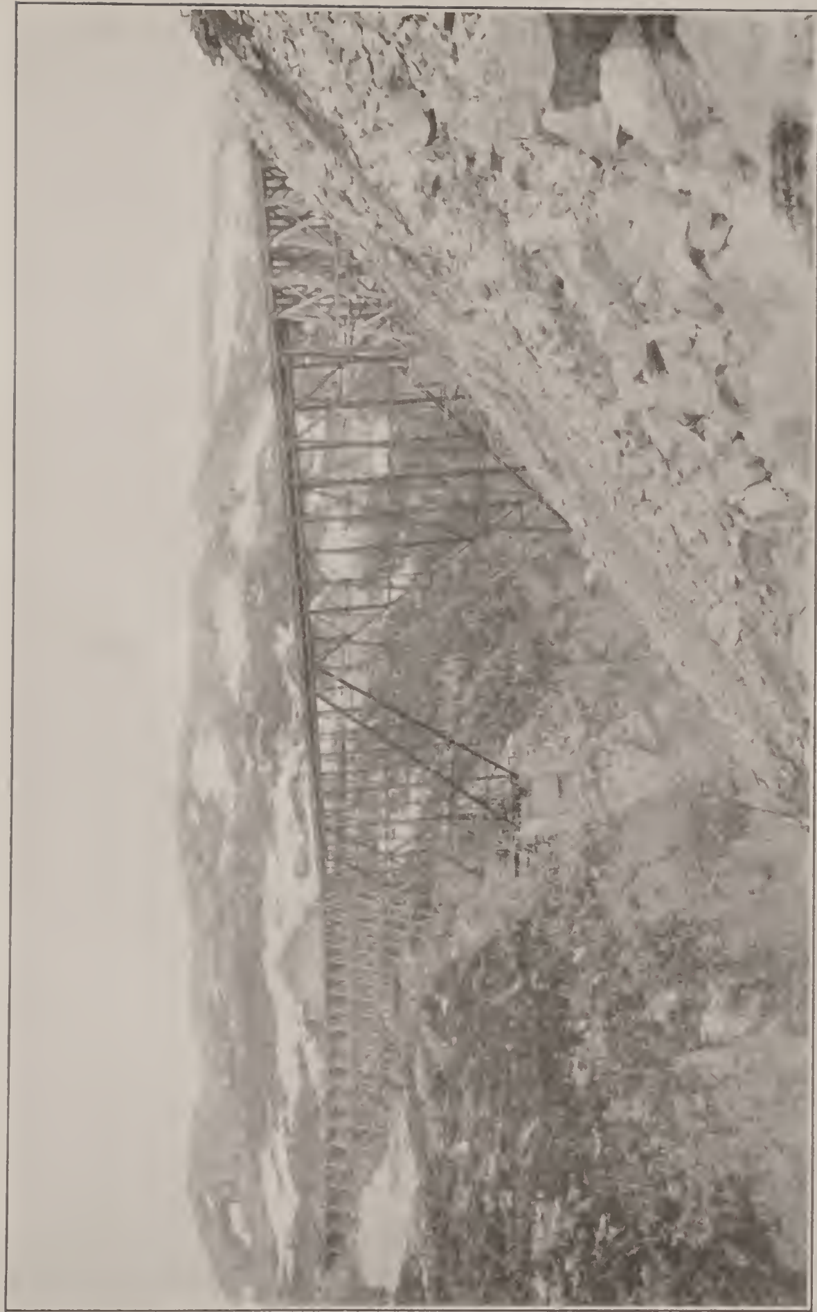
STEEL CANTILEVER BRIDGE, NEAR SUMMIT OF WHITE PASS
